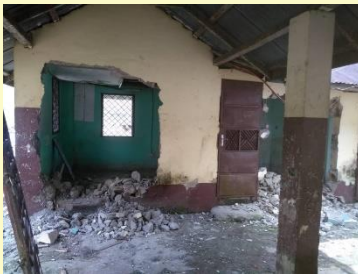
Initial work on the Pa Ngando Project
