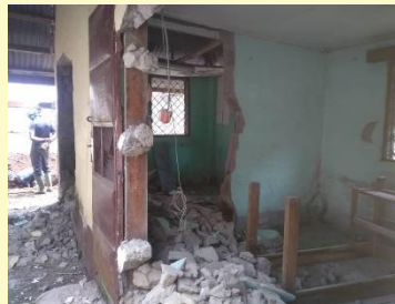
Initial work on the Pa Ngando Project
