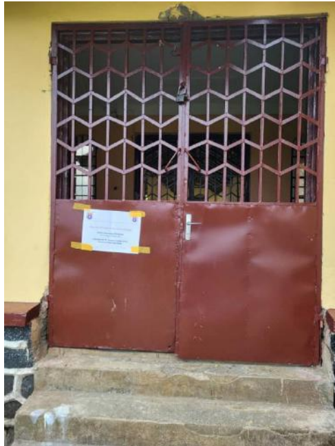
Two side doors at the entrance porch repaired
